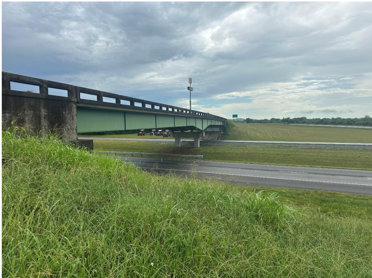
View looking south at existing Epps Mill Road Bridge
